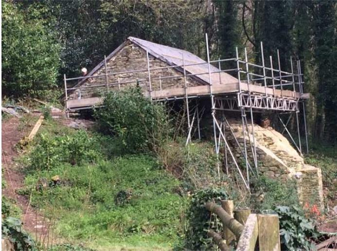
Limekiln reroofing with Lewtrenchard slates
